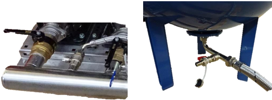
Fig. 1.3a & b Isolation valve on manifold & Flexible hose with drain cock on vessel (non-flow through vessel shown)
